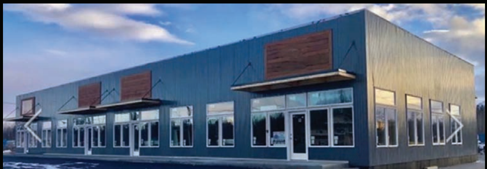
COMMERCIAL SIDING INSTALLED
